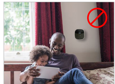
Photo composite showing thermostat on outside wall, which is against building code.
