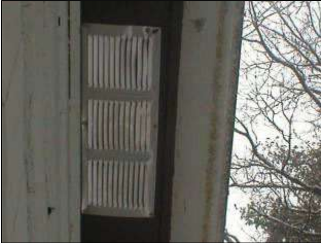
Soffit Vents
