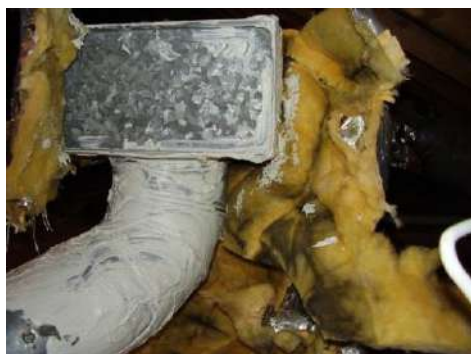
Dirty insulation around joints and seams is evidence of air leakage at duct connections. Duct mastic is applied to seal the leaks and insulation is re-installed.
