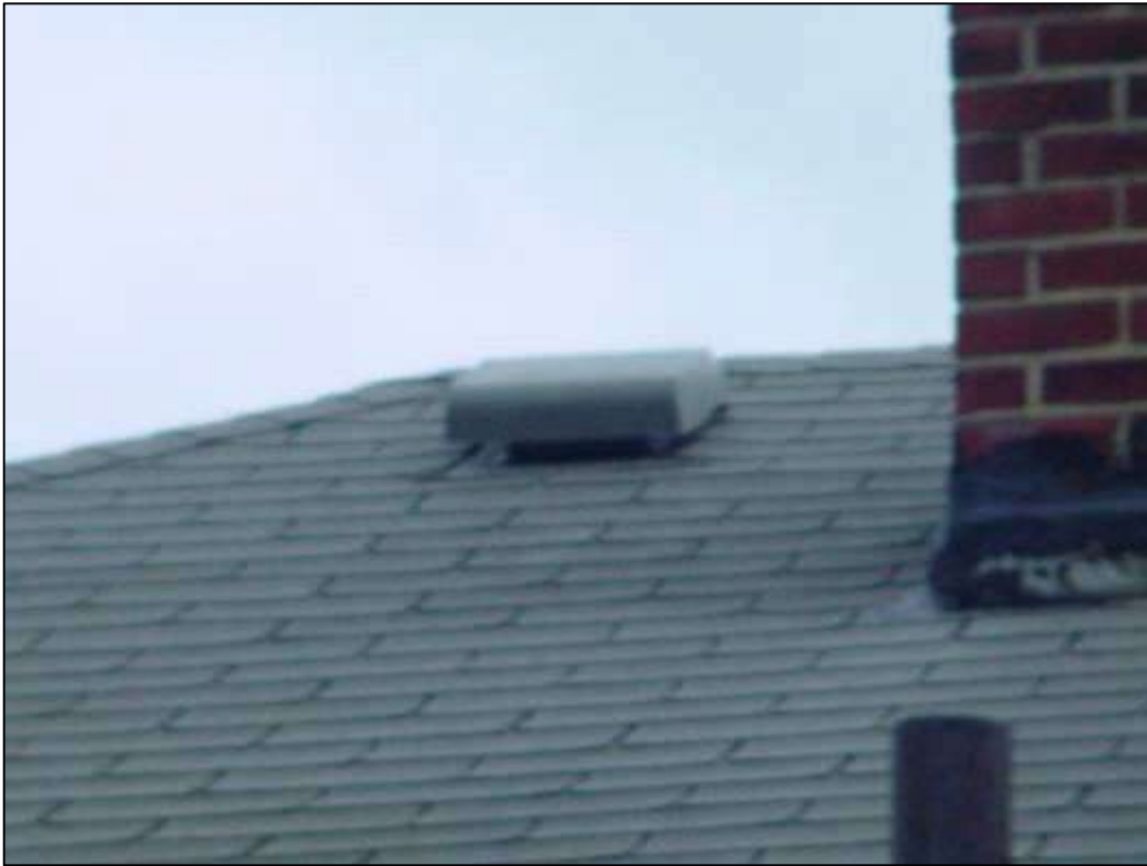
8" roof vent providing .35 sqft of ventilation
