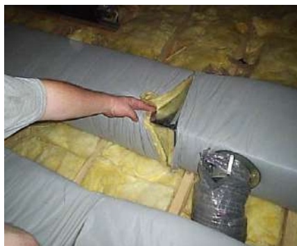
Example of insulation being cut back to expose duct connection that will be sealed with duct mastic.
