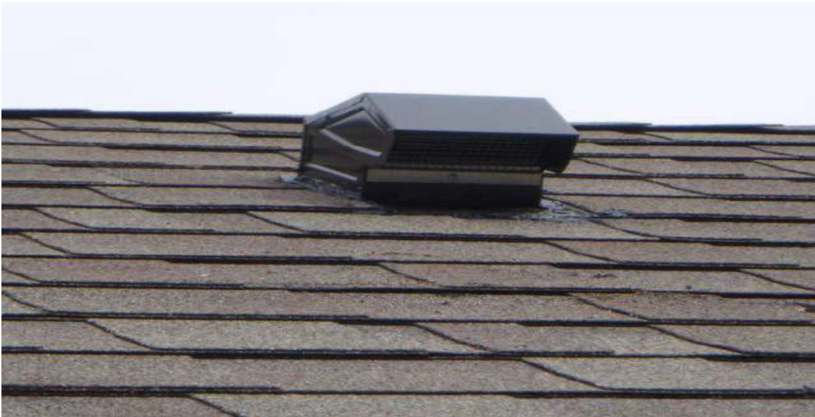
Bath fan vented to roof flapper
