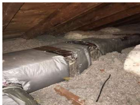
Example of completed duct seal with duct insulation put back in place using program approved materials.
