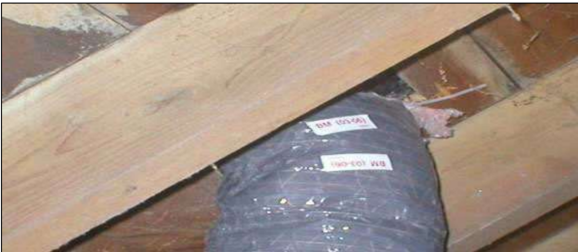
Bath fan vented to roof flapper
