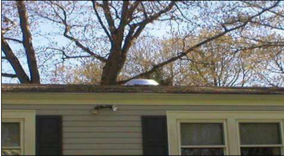
12" roof vent providing 1 sqft of ventilation.
