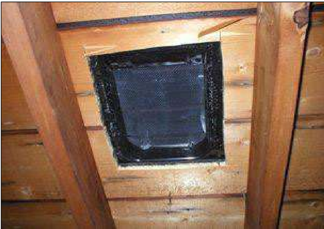
8" roof vent providing .35 sqft of ventilation
