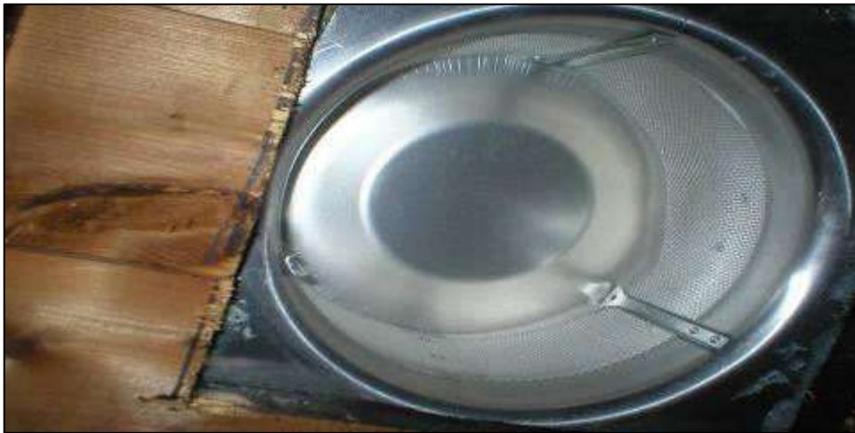
12" roof vent providing 1 sqft of ventilation.
